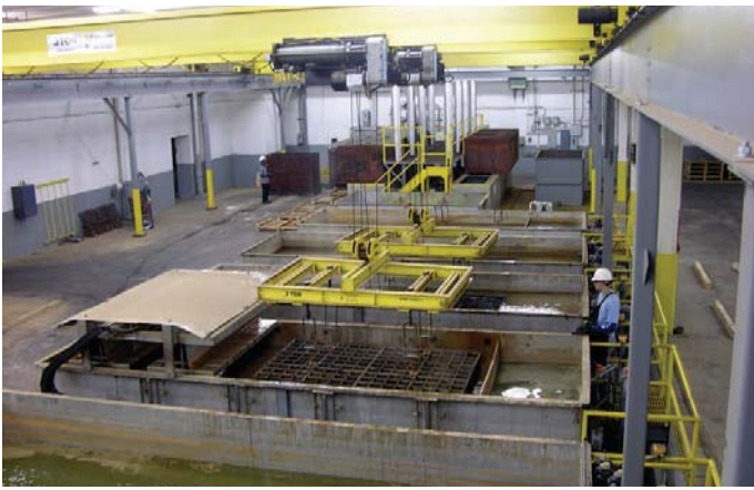
SCR Catalyst Regeneration with Selective Impregnation®
